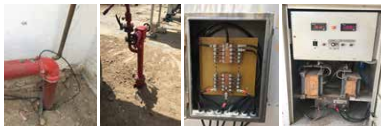
Negative Cable connected to fire hydrant line
