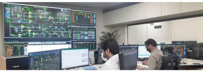
SNGPL's Telecom Department is maintaining a wireless telecommunication network along Company's Transmission right-of-way (ROW) since the inception of the company in 1963. The Department is operating dedicated Digital Microwave Radio Communication System along high pressure gas pipeline network from Sui and Sawan to Peshawar facilitating Voice, Data, Video and SCADA services.
