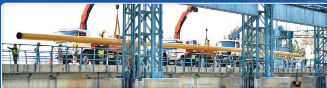
The construction of 18 Inch Diameter Transmission line crossings at Jinnah Hydel and Jinnah Barrage within the domain of Projects Camp, Essakhel, was a challenging and crucial task for SNGPL. However, it was meticulously coordinated among different departments which subsequently resulted in its successful execution.
