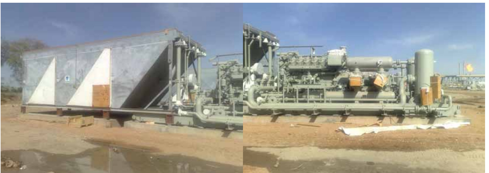
Compressor – Cooler Package Placed on Foundation
