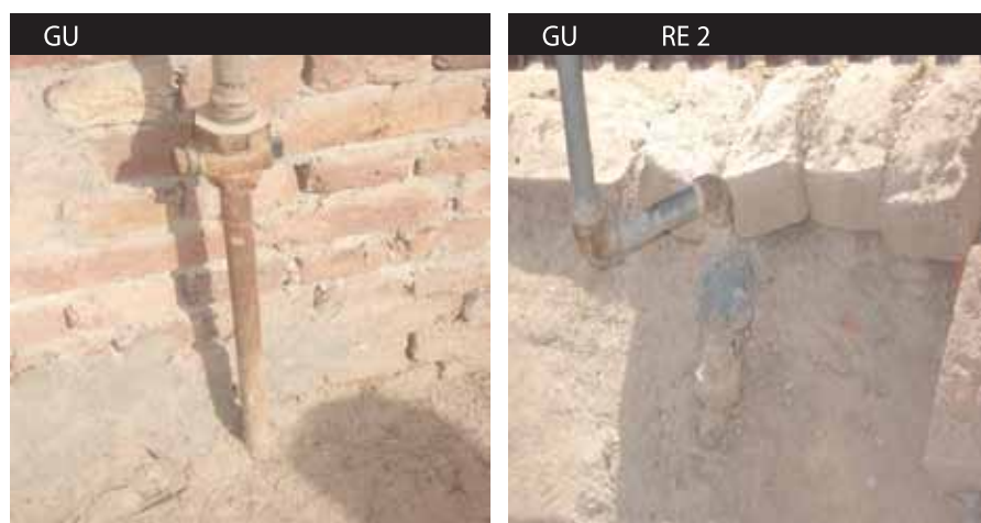
Service line with poor coating.
