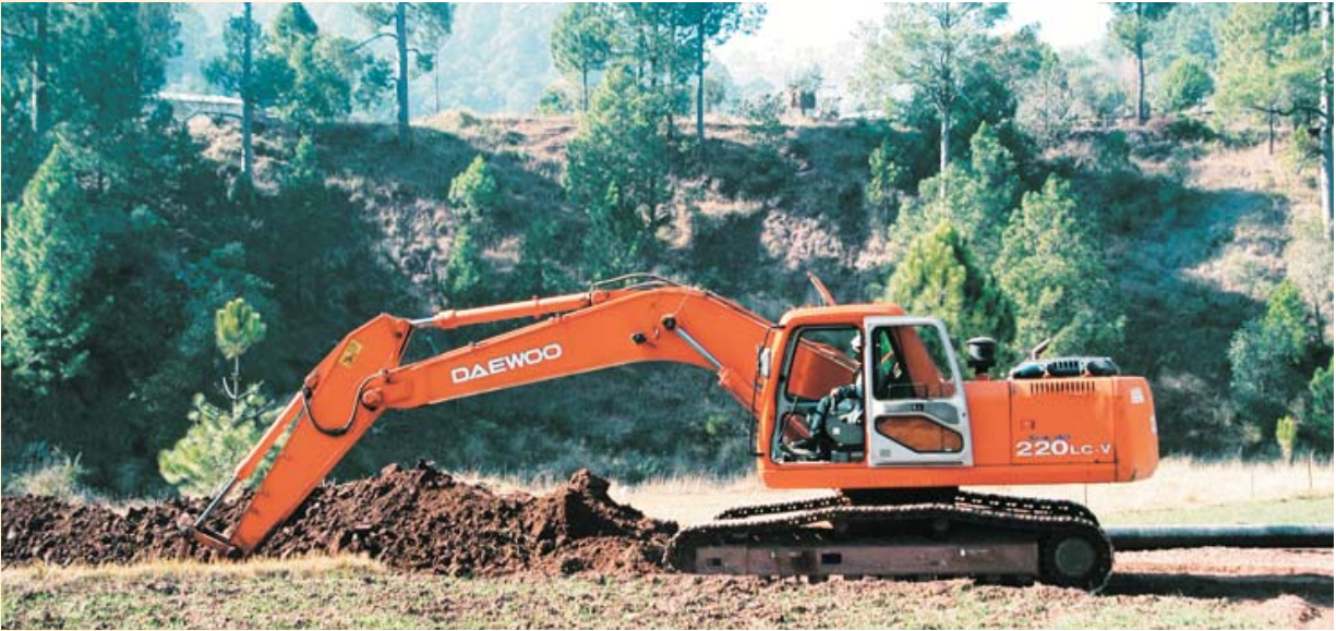
MOVING FORCES - WORK IN PROGRESS - MURREE GAS SUPPLY LINE
