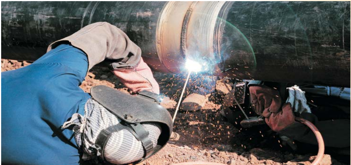
DEDICATED EFFORTS - 12" DIA LINE BEING ENJOINED FOR MURREE GAS SUPPLY PROJECT
