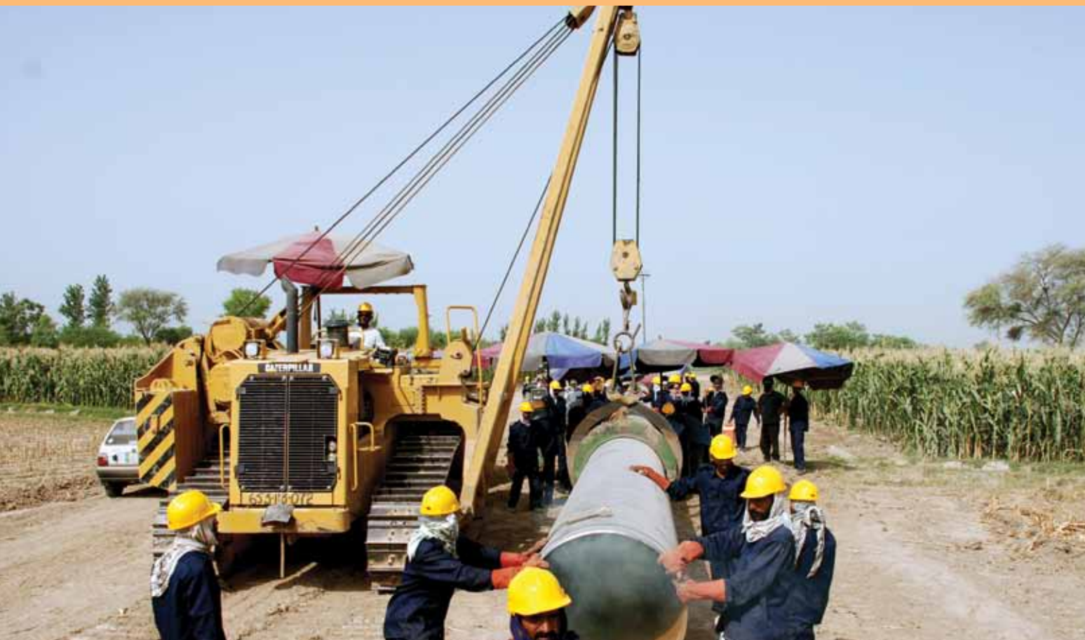
Work in progress of 36" dia Multan-Sahiwal line
