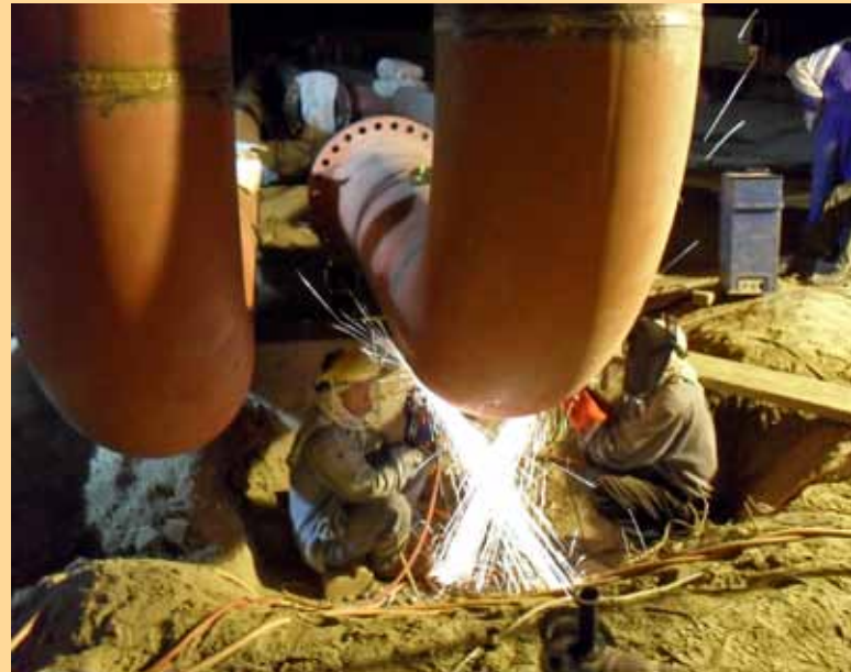
Welding works at Qadirpur field
