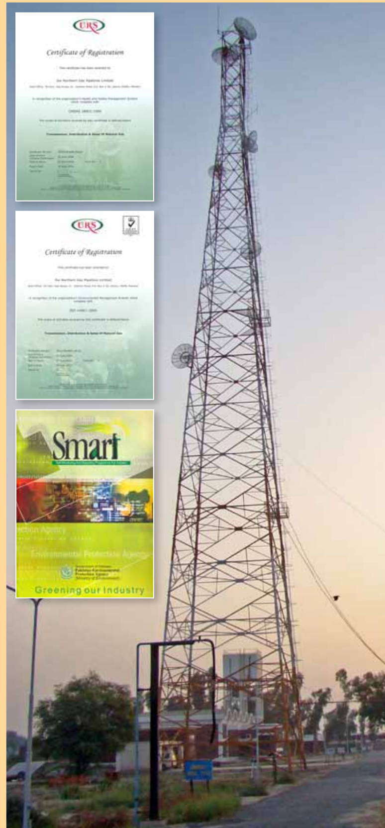
Digital Microwave Communication Tower
