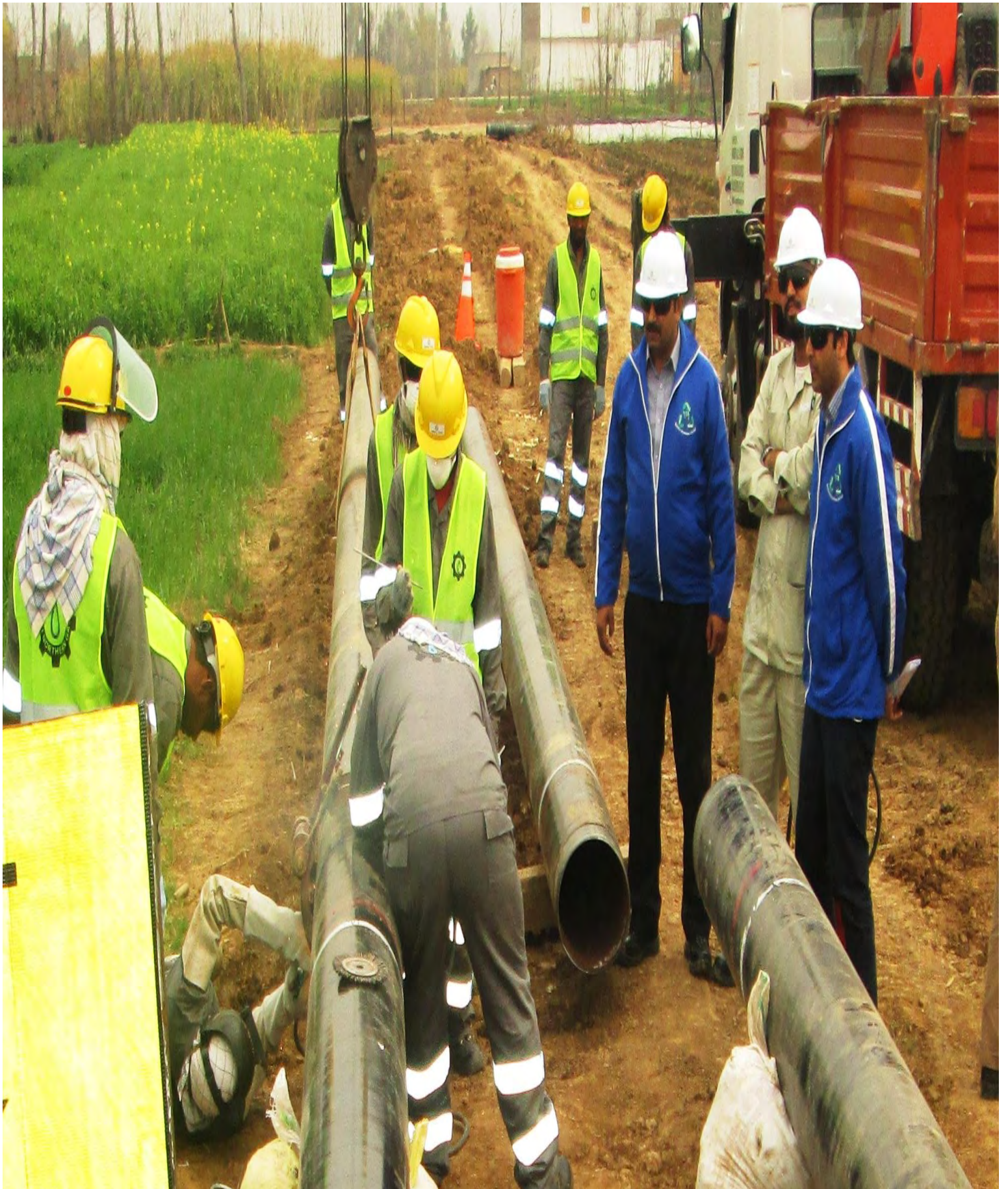
MAINLINE WELIDNG ACTIVITY
