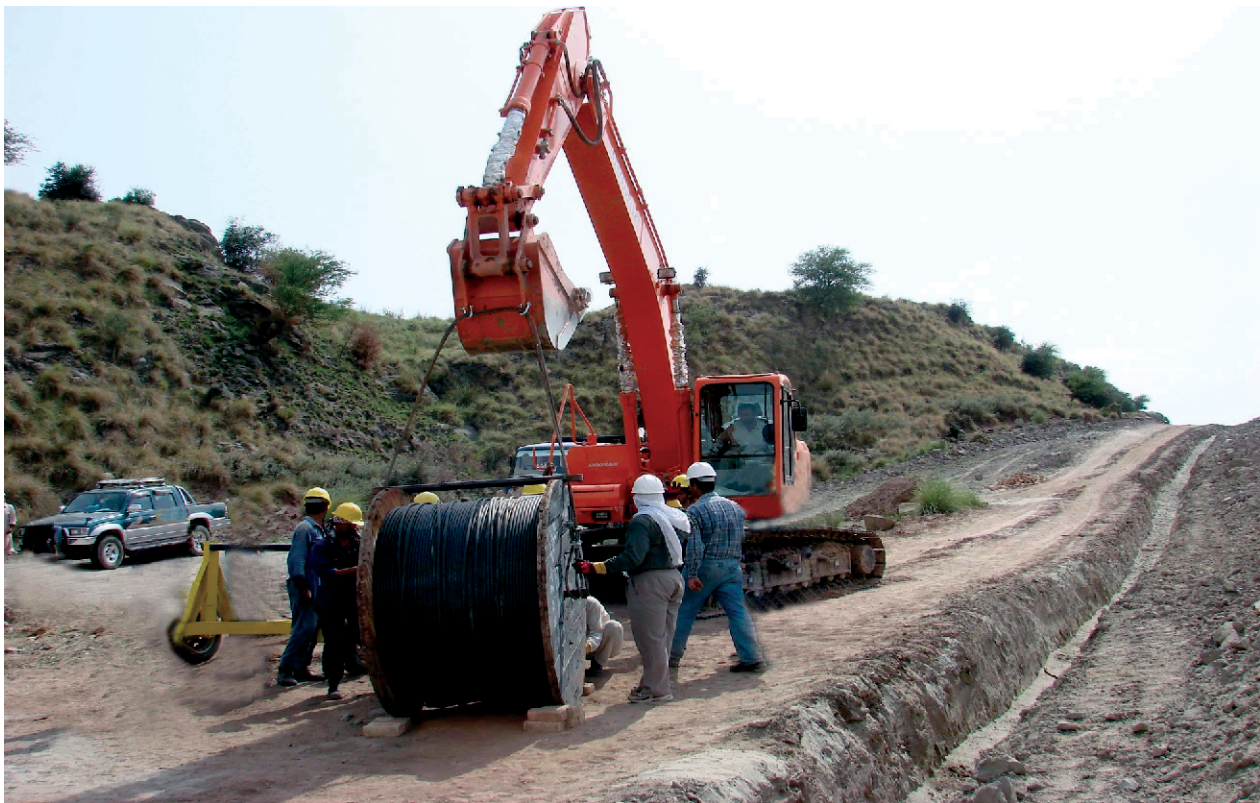
SNGPL Operational Team at the Rocky Terrain of Gurguri Field (Khyber Pakhtun Khwa) for laying Optical Fiber Cable for M/s MOL
