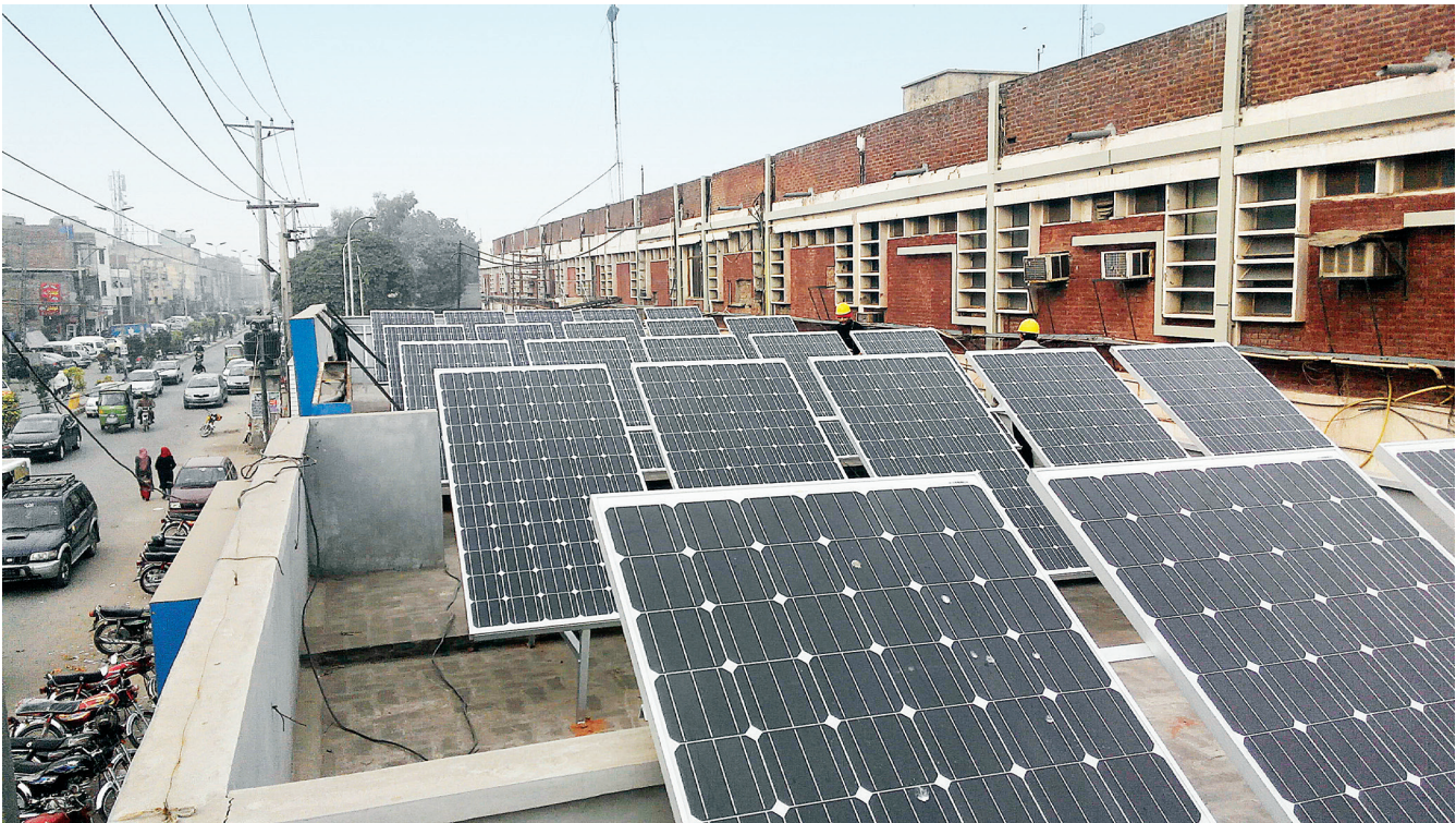
Panels Installed at the roof top of CSC - LHR
