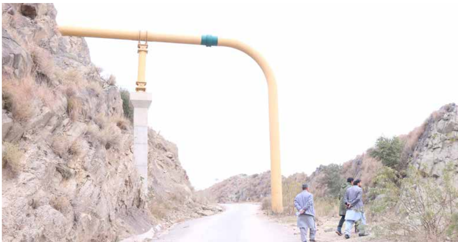
The progress on the project (as on 06.02.2020)
