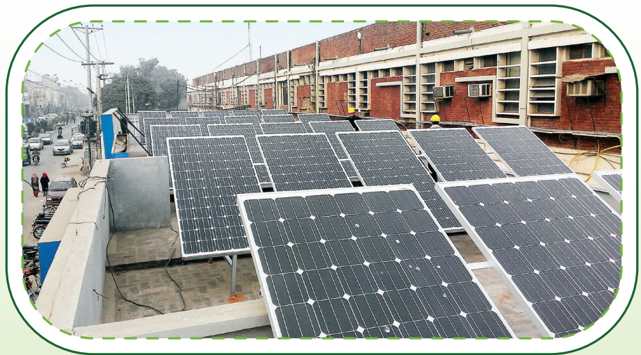
Solar panels installed at the roof top of CSC LHR
