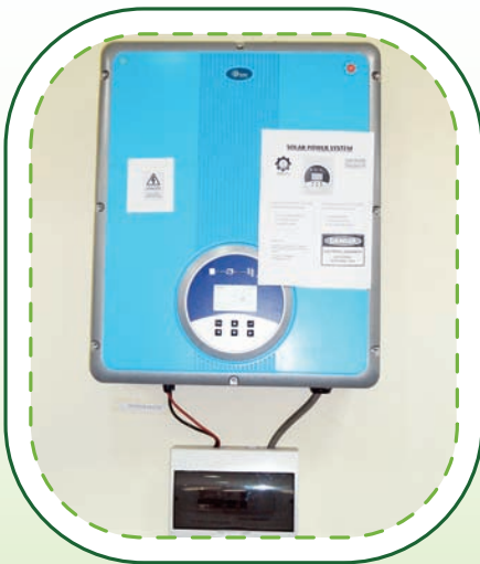
View of Inverter installed in CSC LHR
