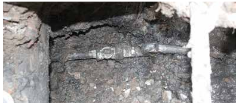
A Bypass installed on 2 gas line being used in Tandoor
