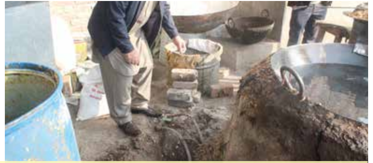
Bypass installed on service line being used in Nimko Frying Unit
