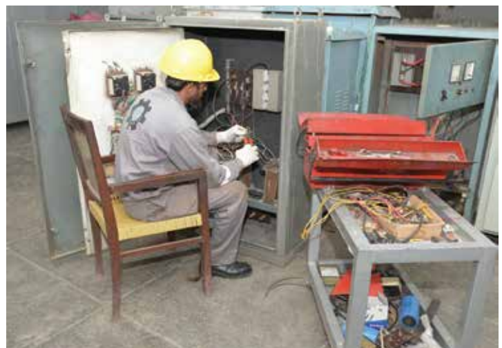
An employee repairing a T/R Unit at the Corrosion Control Center
