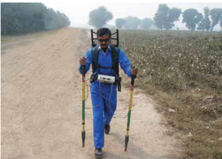
A SNGPL worker doing pipeline survey to assess the CP Level with the most modern equipment.
