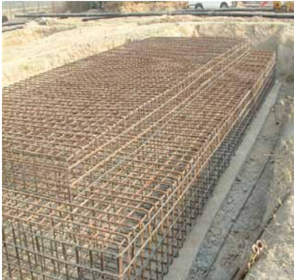
Steel fixing
