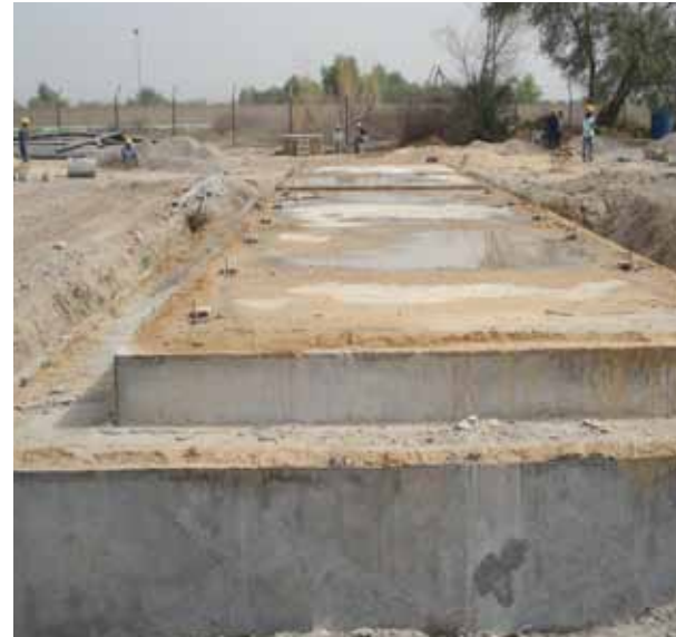
Concrete foundations for compressor cooler unit
