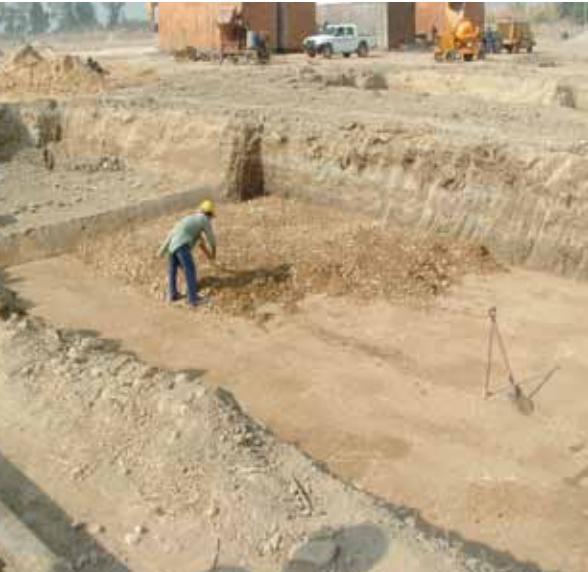
Granular filling & Compaction
